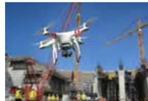
Contractors are using drones to monitor unsafe practices on job sites. A drone with a bird's eye view can provide real-time monitoring of many workers at the same time.
